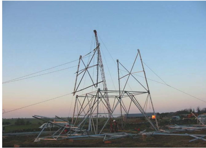
Figure 5.5 Derrick Pole at Tower Base
