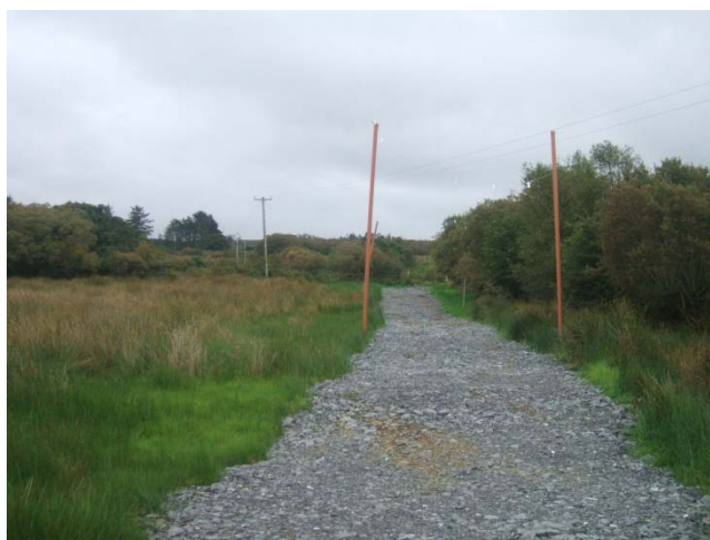
Figure 5.2 Temporary Stone Road
