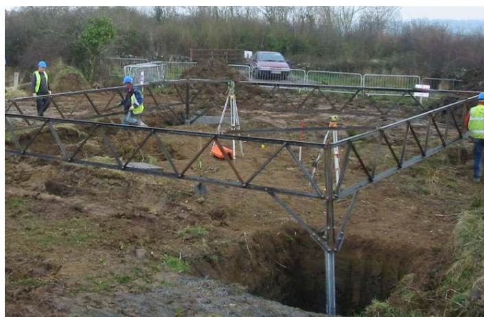
Figure 5.3 Setting Template being prepared for Final Concreting
