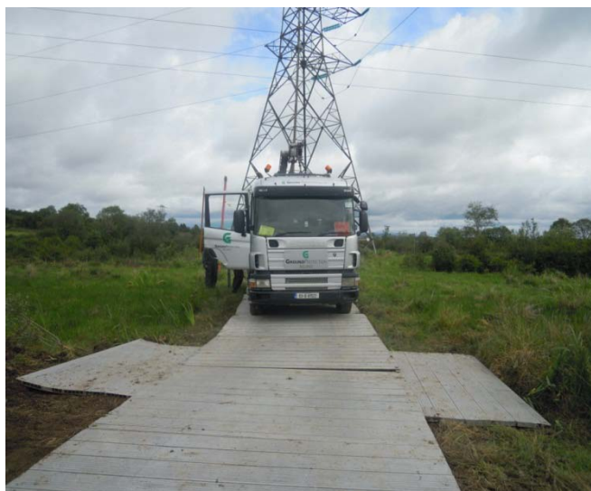
Figure 5.1 Temporary Aluminium Panel Tracks
