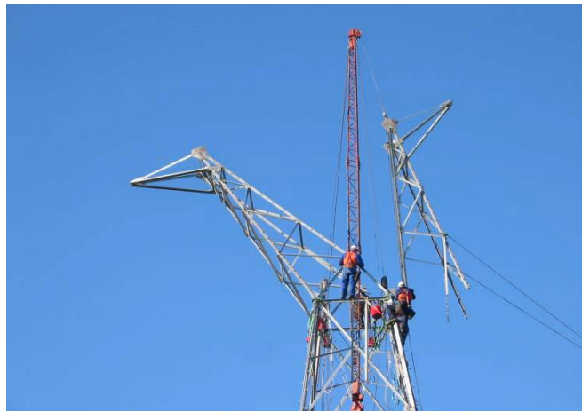
Figure 5.5 Derrick Pole at Tower Base
