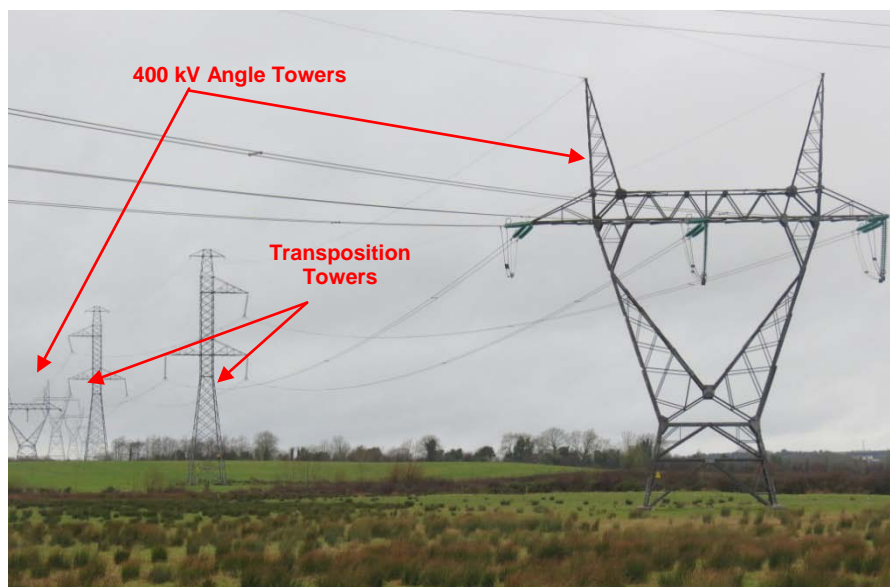
Figure 3.2 Transposition Alignment on an Existing 400 kV Overhead Line
